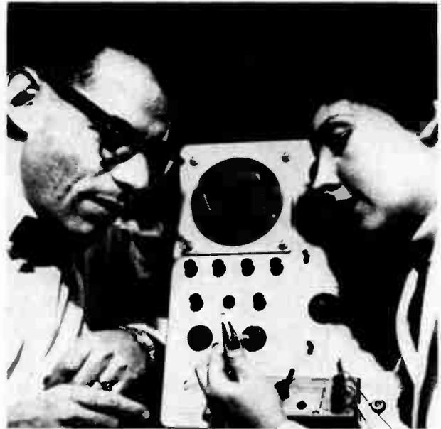
Dr. I. A. Lesk, and laboratory technician, examine one of G.E.'s gallium arsenide tunnel diodes under test.
