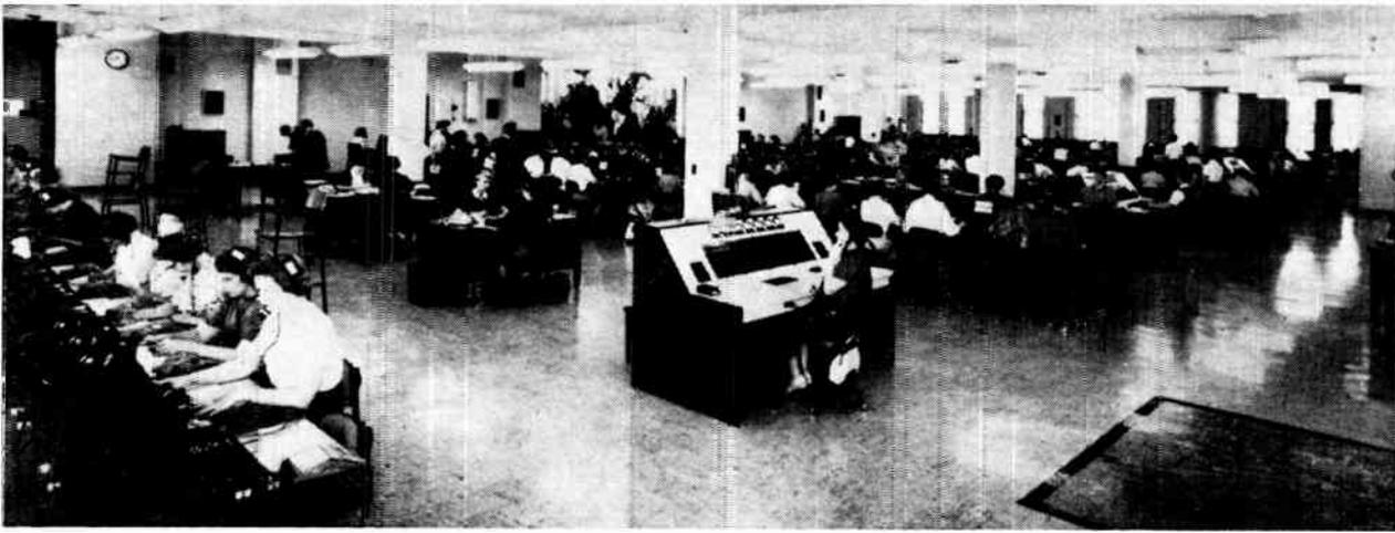
The long distance room in the B.C. Telephone Company's Vancouver headquarters buildings, showing most of the 192-position cordless switchboard. The board went into service in 1959, making it possible for operators to ring any one of some 50 million telephones in North America, without the intervention of operators at the called points.
