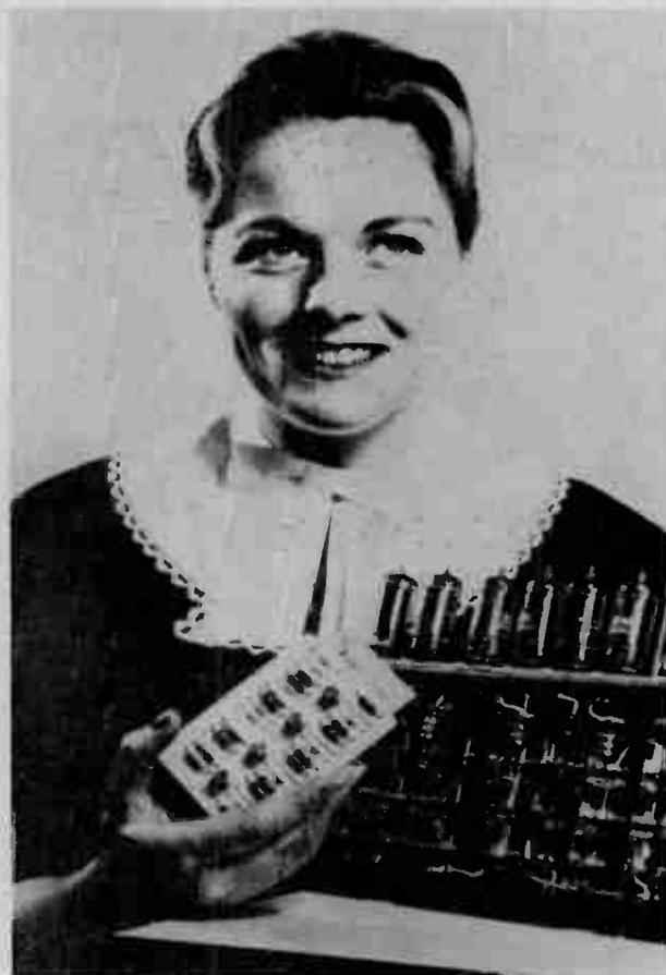
Miniaturization in solid-state data processing equipment can be seen by comparing the printed wiring card (left) used in the new IBM 609 Calculator with a pluggable tube unit (right) used in vacuum tube machines.
