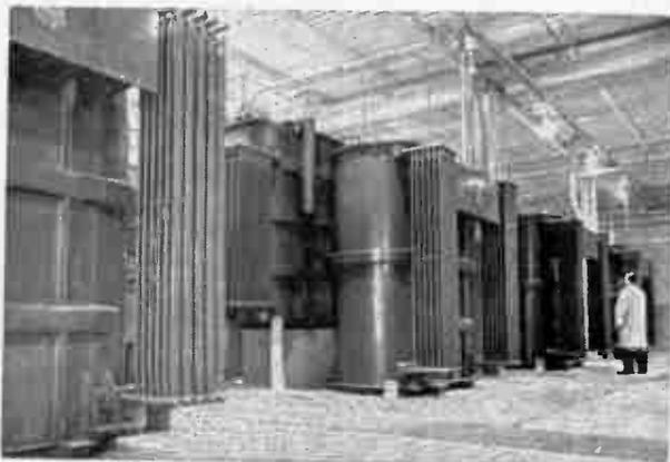
Fig. 2. Bank of high voltage transformers and rectifiers for supplying 120,000 volt DC power to transmitter. Photograph shows units undergoing test at G.E.'s high power radar laboratory, Syracuse.
