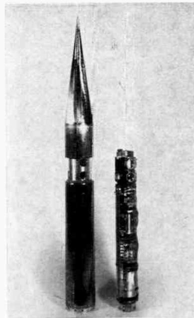
Figure 5. (right) Nose cone structure and instrumented package for Nike-Cajun IGY firings. Package includes two photometers, four radiometers, amplifiers, power supplies, gyro, telemetry and tracking beacon.
