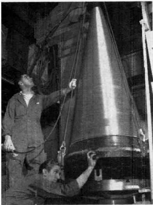
As part of \$500,000 contract fiberglass reinforced plastic radome for CF-104 Starfighter is positioned on grinding equipment at Brunswick of Canada's Dixie plant.
