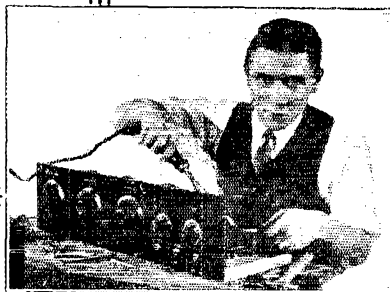
Front View KD-50 Neutrodyne Being Assembled
