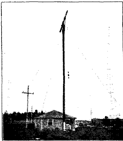
THE ANTENNA SYSTEM AT 2XAF
