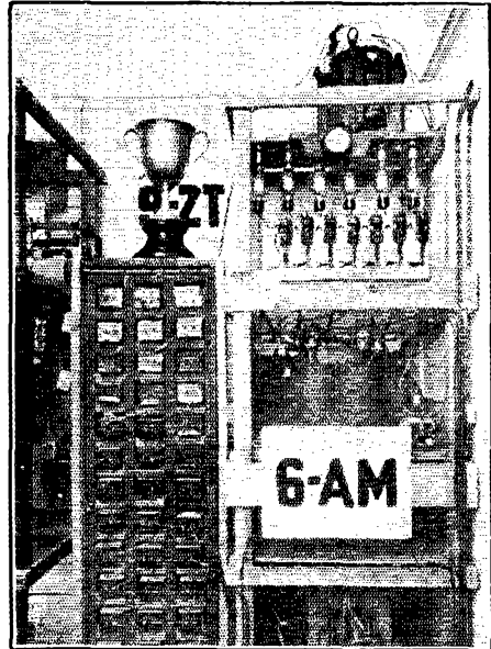
THE FILTER BANK AND POWER PANEL. The rather impressive condenser bank is not often used. It is made of many low-voltage old-style condensers and has a total capacity (with present connections) of 1/3 μf, which is ample to turn the note of this station into "pure d.c.", showing the great ease of filtration. In the power panel we have from top to bottom, 3-k.w. transformer used for Kenotron filament supply, bank of rectifier tubes, one group of high voltage transformers, some chokes, second group of high-voltage transformers. The cup and the 9ZT card are Minneapolis souvenirs.
