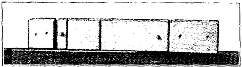
THE TWO BLOCKS USED IN FORMING THE CORNERS
