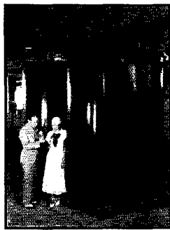
It's a boost of a few decibels from the tiny microphone transformer, scarcely visible in the OM's hand, to the mammoth double-unit Class-B output transformer in the background. This transformer, weighing upwards of 50 tons, has an audio output capability of 400 kw., as is required for modulating 100 percent the Class-C amplifier operating with 800 kw. average input. Besides its necessary ingredients of iron and copper, the transformer contains 1400 gallons of oil for cooling.
