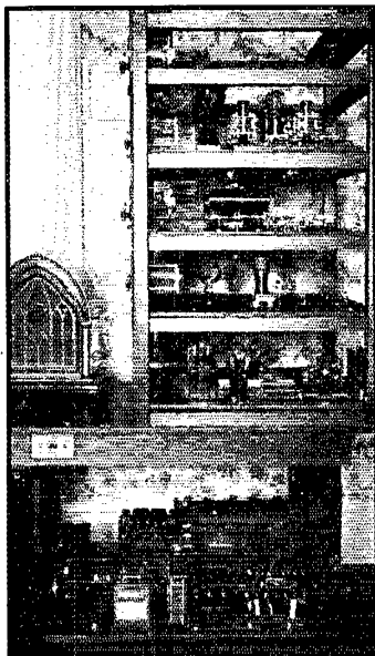
THE SIDE VIEW OF THE TRANSMITTER, SHOWING ALL POWER SUPPLIES LOCATED ON A SHELF AT THE BOTTOM, WITH THE MODULATOR SHELF ABOVE
