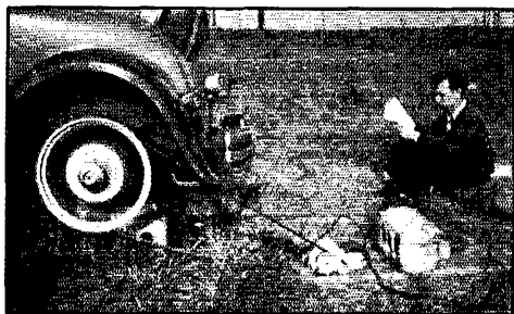
W9SUJ/9 KEEPS AN EYE ON THE LINE VOLTAGE DURING THE 27-HOUR CONTINUOUS RUN
