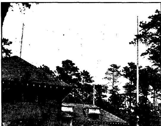
PART OF WICCZ'S ANTENNA SYSTEM
