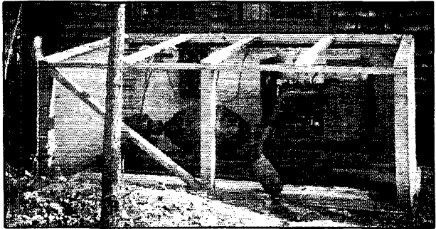
THE HIGH-VOLTAGE GAS-ENGINE-DRIVEN GENERATOR WITH COVER REMOVED FROM THE HOUSING
