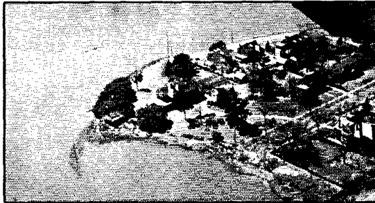
The high poles on the point and along the water's edge belong to the antenna system at W3EMM. W3EMM's is the house on the point.
