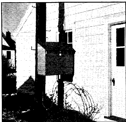
The "flat-top" rotatable antenna is turned by a motor and reduction system housed in the "dog house" mounted at the base of the supporting pole.
