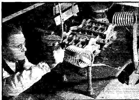
Power is off and it's safe to tangle with the antenna network of 100-kw. WGE0.
