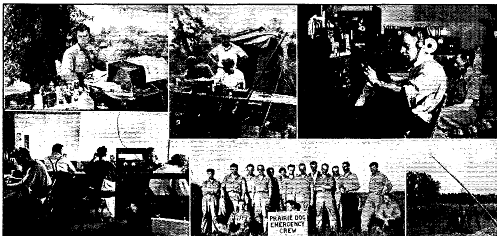
Upper left: Three rigs were used by the W5FOP/5 group. Pictured is W5FOP at the key of the 14-Mc. unit. The receiver is an FB7 with preselector and the transmitter the popular 6L6-807 combination. Upper center: Members of the Rubber City Radio Club operated W8UMJ/8 in the one transmitter classification. Left to right: Bob Lyman, W8NXI, W8TOL. Upper right: The Cuyahoga Radio Association, W8URA/8, were situated in a 25-foot trailer for their F.D. work. W8WV (l.) and W8EBJ (r.) are shown keeping things humming. Lower left: Six simultaneously operated units were used by the St. Paul Radio Club, W9KYC/9. Seated at four of the positions are: W9QDF, W9QPL, W9OCN (monitoring operator), W9YCR and W9QPG. Lower center: Sixteen of the eighteen members present for the Prairie Dog Emergency Crew's participation in Field Day. Their station, W9JU/9, placed first in the four transmitter classification of the non-club groups. Lower right: Members of the Norfolk Radio Club hard at work raising a pole to support antennas at W3BEK/3.
