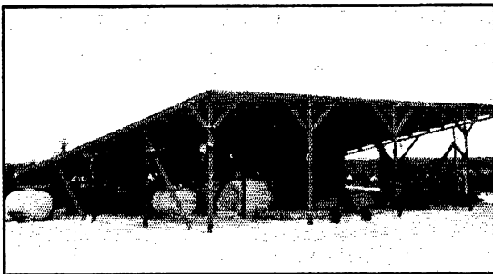
Drinking water was collected on the roof of this shed and fed into drums through a trough.
