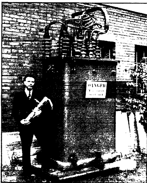
W8UNS alongside the 100-kva. power transformer. The bottle is an 859, rated at 40 kw. input. Two of them are used in the cyclotron oscillator.
