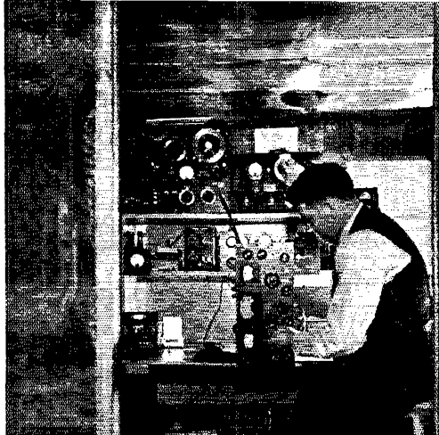
Shielded test booths are an important part of a modern radio plant. Outside QRN cannot be tolerated while critical adjustments are being made. Grounded copper screen completely encloses each test room.
