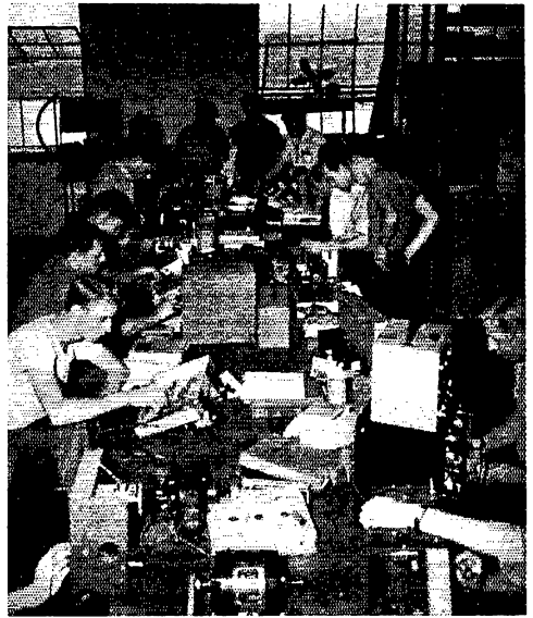
JRT class at work on a transmitter project at the Lafayette Trade School. One group builds r.f. unit while another constructs the modulator.
