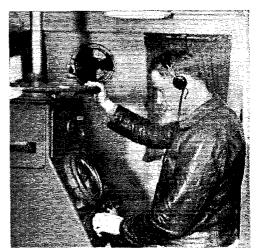
The navigating officer takes a directional bearing on the radio direction-finder. One hand operates the handwheel controlling the rotatable d/f loop above the deck while the other adjusts the magnetic balance control.
