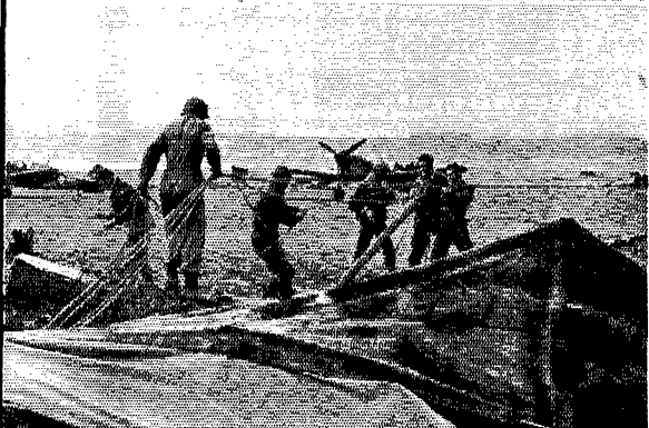
Signal Corps troops set up a mobile message center at an airdrome in North Africa. Top — Members of an aviation engineers unit dig a canvas-walled shelter for the SCR-299 near Youka les Bains in Algeria. Center — The radio truck is driven into its shelter and camouflage netting draped over the top. Above — Additional camouflage completes the job. Right — Mobile signal battalion message center in Tunisia.
