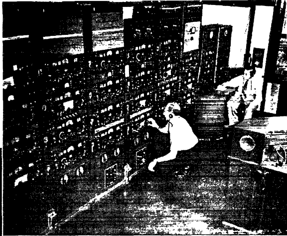
Above—The monitoring officer in the foreground adjusts the receiver of a station to be monitored a few minutes later. The officer in the background scans the ether for new or unknown stations. Left—Instantaneous frequency checks may be made at any time by connecting this special switch.
