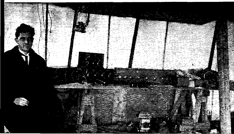
Interior of the tent "ham shack" used by Mr. Godley. Inspector D. E. Pearson, checking operator, is shown seated alongside the makeshift receiving position, the lantern and oil stove.
