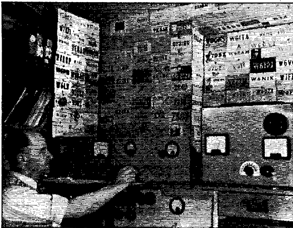
First ticketed in 1938, GW4CX has since made quite a splash on 14 and 28 Mc. Operator T. W. Coplestone is shown in the pilot seat. Transmitter: 6V6, 807 and p.p. PT15s; receiver: BC342 and converter for 28 Mc.; antennae: long wire and 3-element beam. Having worked a thousand Ws since the war, GW4CX nevertheless managed to snare 120 countries.
