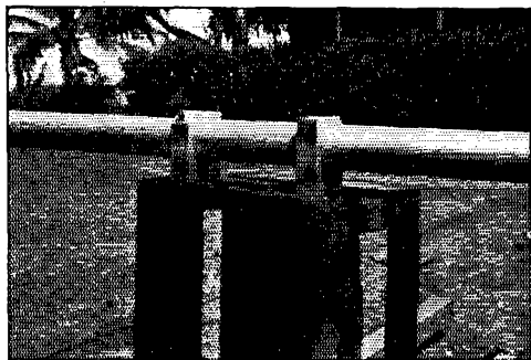
The boom is held to the mounting plate by two solid pieces of cast aluminum.
