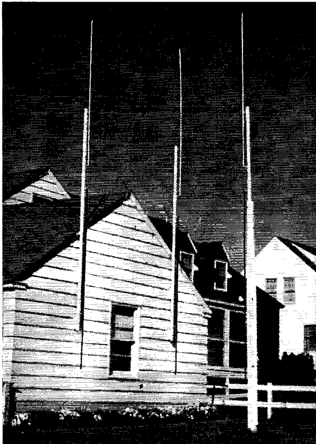
The phased vertical antenna system installed at W2OOM. In this arrangement, only one small mast is required.
