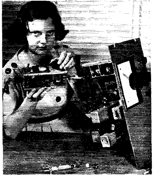
The second YL to get an Extra Class license, so far as we know, W4MKP operates 20, 40 and 80 c.w., using only gear which she has built herself — receiver, and even coils, included. She is shown here aligning her superhet. (Photograph courtesy Prof. S. A. Coons, M.I.T.)
