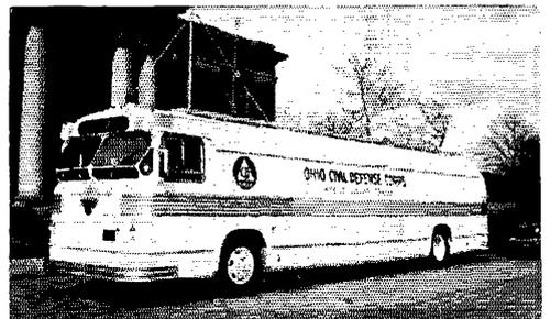
This mobile communications control center belongs to Ohio State Civil Defense and was on display at the Ohio State Fair last August. In addition to the usual array of telephone, teletype and commercial radio gear, it has four amateur operating positions using Collins, Johnson and General Electric gear. Power is provided by a 15-kw. Onan gasoline-driven generator. W8FYW Director of Communications for Ohio CDC, has charge.
