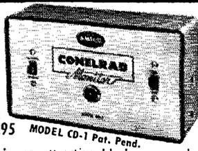
Completely enclosed in an attractive black case and brushed copper panel with block lettering, the AMECO Conelrad Monitor converts any receiver having AVC, into an effective conelrad alarm system. When the broadcast station goes off the air, a loud clear tone is immediately sounded in the receiver. The AMECO Monitor is a complete electronic audio alarm. There are no buzzers or relays.
