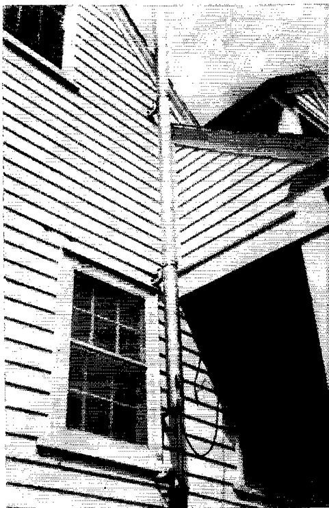
The mast is secured against the side of the house on brackets made of standard fittings.
