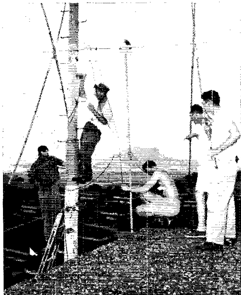
Just about all set for FD action is this cubical quad being put together by the Caribbean Air Command MARS RC, KZ5AF/KZ5. Handling its construction are from left to right: KZ5s RB, BS, RR, LL, and W3VOC.
