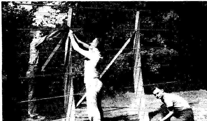
Wiring on the hardware-cloth reflector. Workers are, left to right, Dave Walker, Vern Robertson, W1EGE, and Southard Lippincott, W1DDN.
