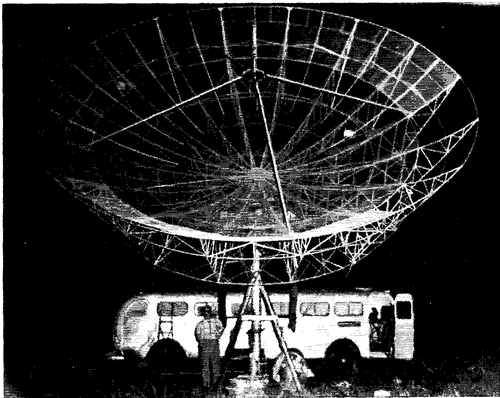
W8LIO's almost-completed 26-footer for 1296 Mc.
