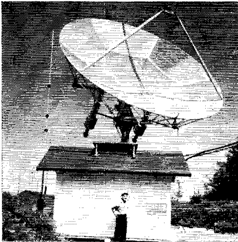
Above, the antennas at KH6UK and W1BU. KH6UK got his 28-foot Kennedy through MARS, while the eighteen-footer at W1BU came from surplus. Sam's dish tracks automatically. Below, the transmitters. Both used one-kw. kylstrons by Eimac.
