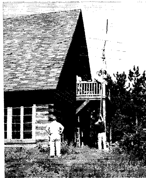
Up they go! The 6- and 2-meter beams of WA2IOG/2 are hoisted to their position on a building of the Rutgers Experimental Farm.
