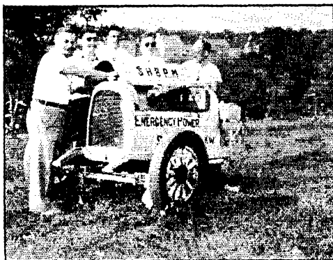
This was typical of Field Day power sources in 1938. This one was used by the South Hills Brass Pounders and Modulators (Pittsburgh, Pa.) and delivered a total of 4 kw.
