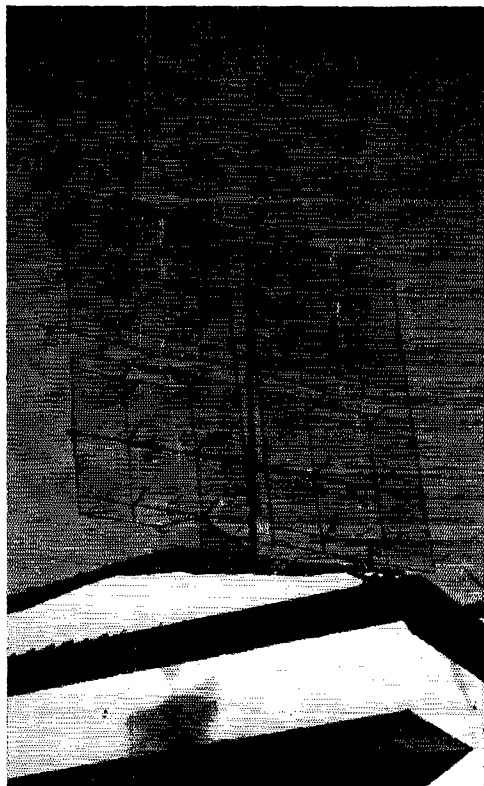
OH1NL used this 24-element phased array in front of a screen reflector for his end of the record-breaking 144-Mc. moonbounce contact with W6DNG. The whole assembly is mounted on his rooftop and is tiltable to +30 degrees above the horizon.
