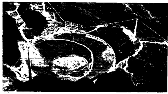
1000-foot reflector at the Arecibo Ionospheric Observatory, used in the 420- and 144-Mc. moonbounce tests.
