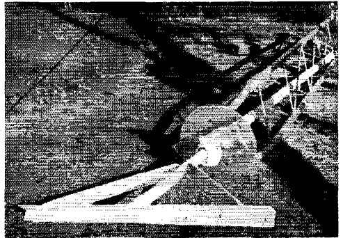
Top section of the tower before mounting, with the bearing, antenna yoke and top section of the drive shaft in place.
