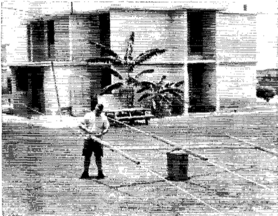
The author lashes a bamboo support in place. The 2 \times 2 crossarms have already been nailed to the 2 \times 4 boom.
