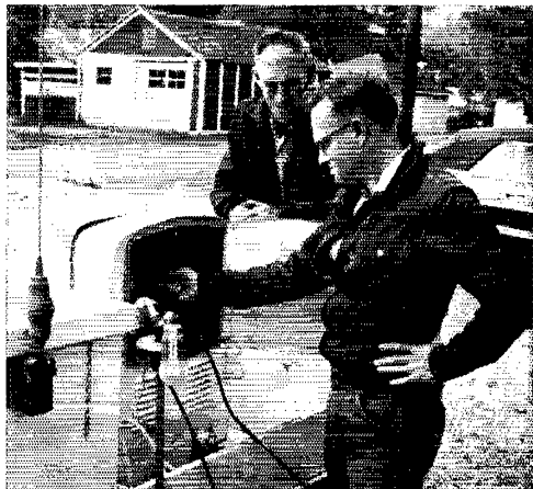
Many AREC groups made the test more realistic by using emergency power. Here K9SGB adjusts the generator being used by the Randolph County, Ind., group while WN9MPL looks on.
