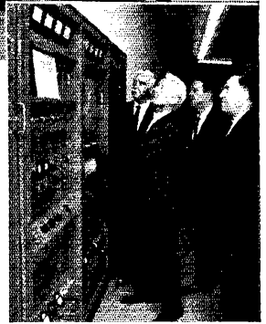
Mr. Peter Viezbicke, Bureau of Standards' Installation Engineer, adjusts one of TMC's 40 kW transmitters shortly after the first signals were broadcast from the new Ft. Collins facility at 0000 GMT, 1 December.
