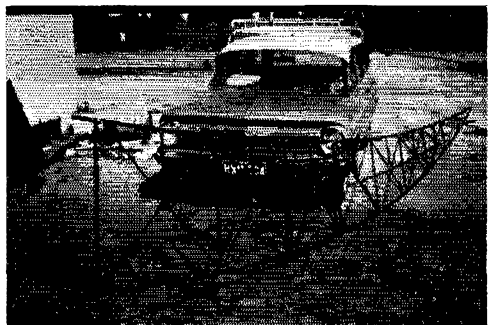
This is one of the more than 20 steel tubing trusses being used in the 50-foot dish at VK3ATN. The 20-foot long trusses weigh 30 pounds each and are within 1/8-inch tolerance of a parabolic curve.
