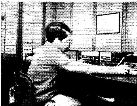
Missouri's 13-year-old WNØRVR breezing along on a TO keyer en route to 5,950 Sweepstakes points. Tom's FB setup also includes a Drake 2NT transmitter, 2C receiver and a 14AVQ vertical.
