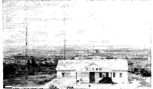
Pittsburgh is the Steel City, and it would appear as though a hefty amount of that steel winds up as antennas for Steel City ARC's W3KWH . At right is a view of the shack (shack?); looking west, we note (left to right) a modest 64-element collinear array for 144 MHz, an 11-element beam for 50 MHz, and a 32-element job (up about twenty feet) for 432 MHz. At left is a neck-crane closeup of the 2-meter monster.
