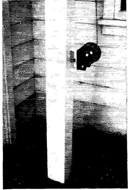
A winch mounting is welded to the 6-inch column at a convenient level above ground.
