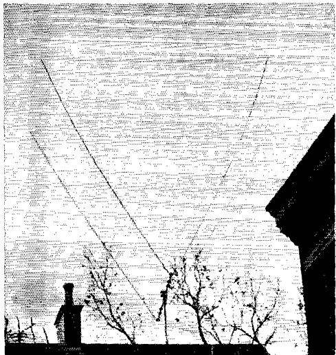
Here is our roof mounted 20-meter Delta Loop beam that is now undergoing a series of tests.
