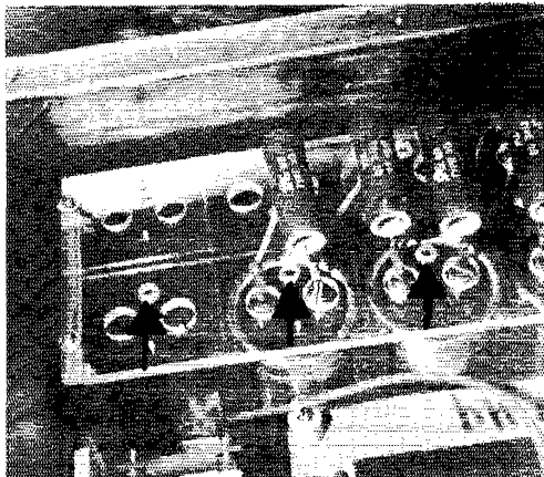
Fig. 4—A view of WB2ZQH's partially constructed power supply illustrating the practice of providing relief holes for the safety vents of computer-grade capacitors.
