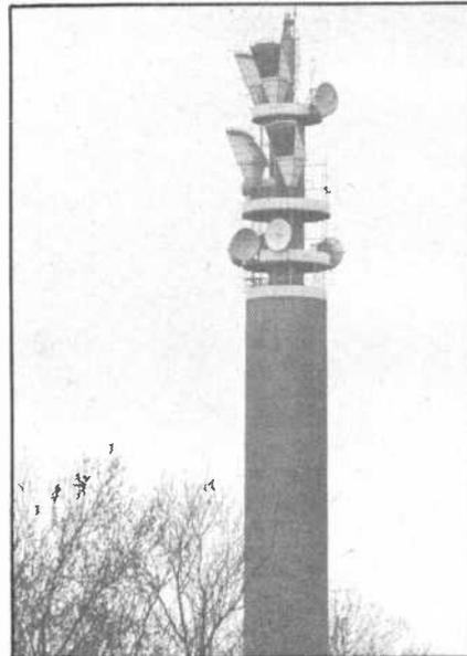
Height is important for VHF, UHF and microwave antennas — hence the tower!
