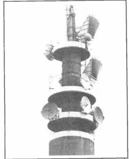
*Above: It looms large and is imposing, the Stokenchurch antenna tower. But it's only a repeater for the London Post Office Tower, handling microwave trunk calls to and from the west of the country.*
