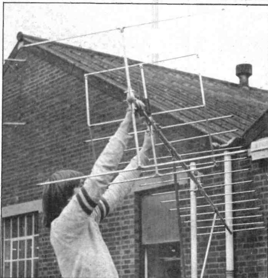
Top: Jaybeam's TB3 is a Tribander measuring 51mm boom diameter, and 420cm boom length. This one costs £165 but retains a peak gain of 8db and maximum input power of 2kw PEP. Above: The PBM14/2m is a panabeam yagi with a length of nearly six metres.
